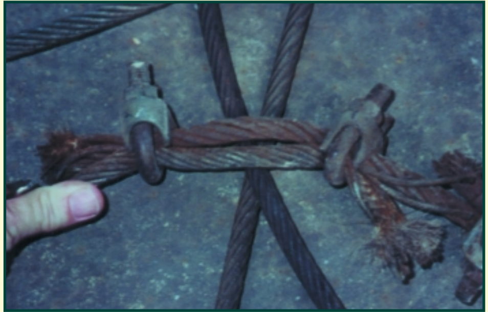
Failure of manlift cable at location of the unsafe repair.
