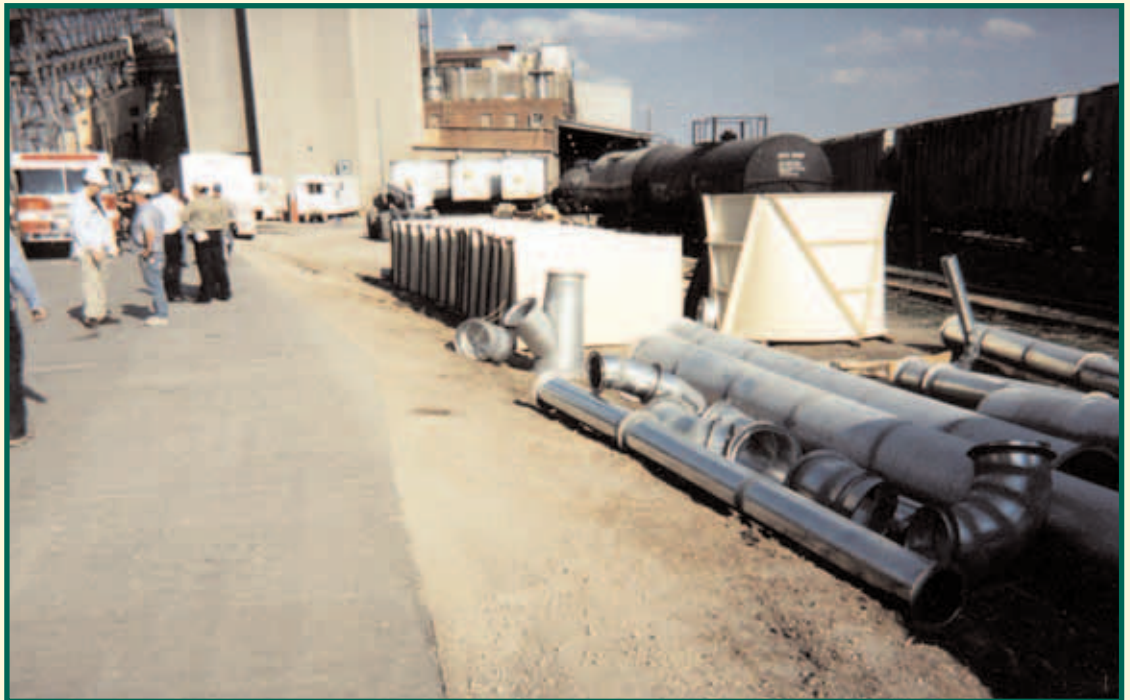
Staging area at Grain Processing Facility.
